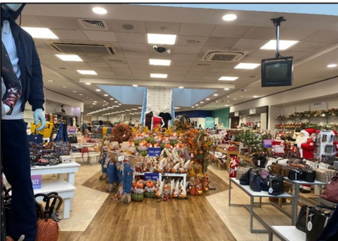
Escalator between GF and FF at GF level
