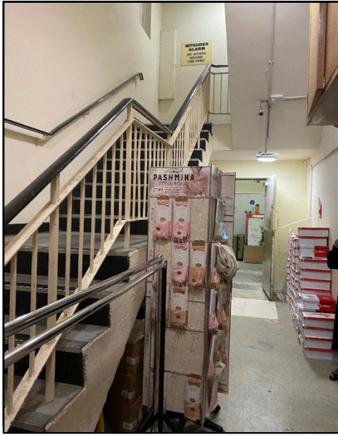
Rear Fire exit Stairs
