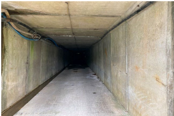
Water Treatment Works
