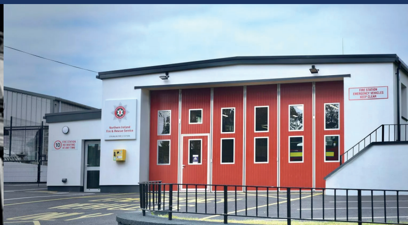
Refurbishment and Extension at Crumlin Fire Station, Source Northern Ireland Fire and Rescue Service
